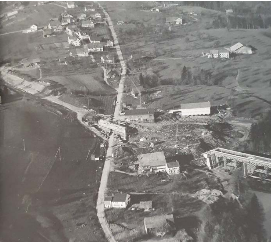
Nationalstrassenbau 1960 N3 in Horgen
